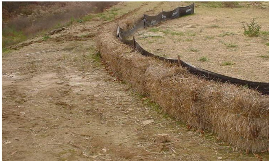
FIGURE 4.2 EROSION CONTROL USING HAY BALES, PHOTO PROVIDED BY GOOGLE
